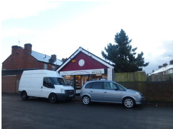
Photo taken facing south towards the principle elevation of the application site
